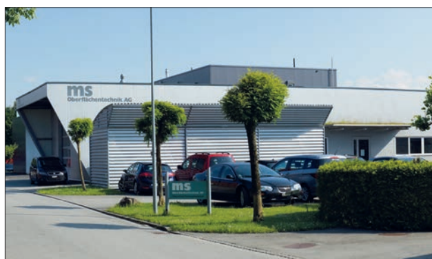
Balgach, Switzerland facility
